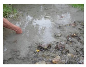
by hand. The washed out area immediately downstream of the breached sedimentation basin was seeded and stabilized with hay. Finally, hay bale sediment barriers were installed at strategic locations along the affected tributary as well as the main stream channel to prevent the degradation of additional spawning beds downstream of the areas already affected.
