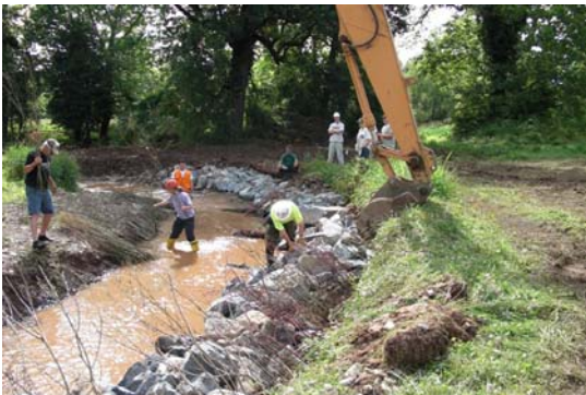
Meander #2: During active construction
